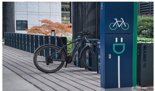
FIGURE 5. E-bike charging station
